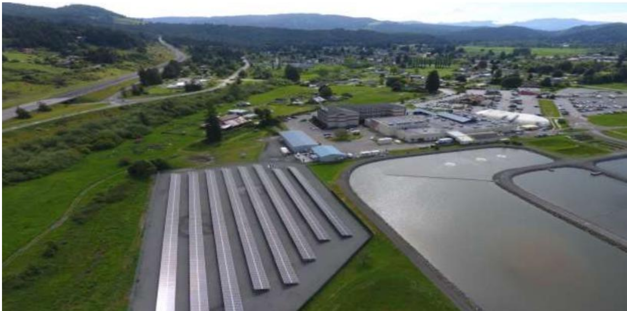
FIGURE 16 THE BLUE RANCHERIA MICROGRID PICTURE PROJECT OVERVIEW
