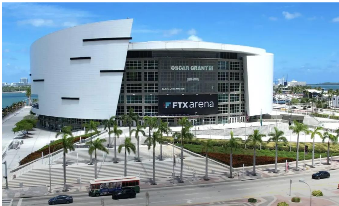
Figure 14. FTX Arena in Miami.
